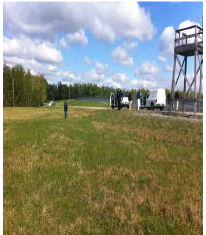
Southeast cap looking west. Survey tower in background.
