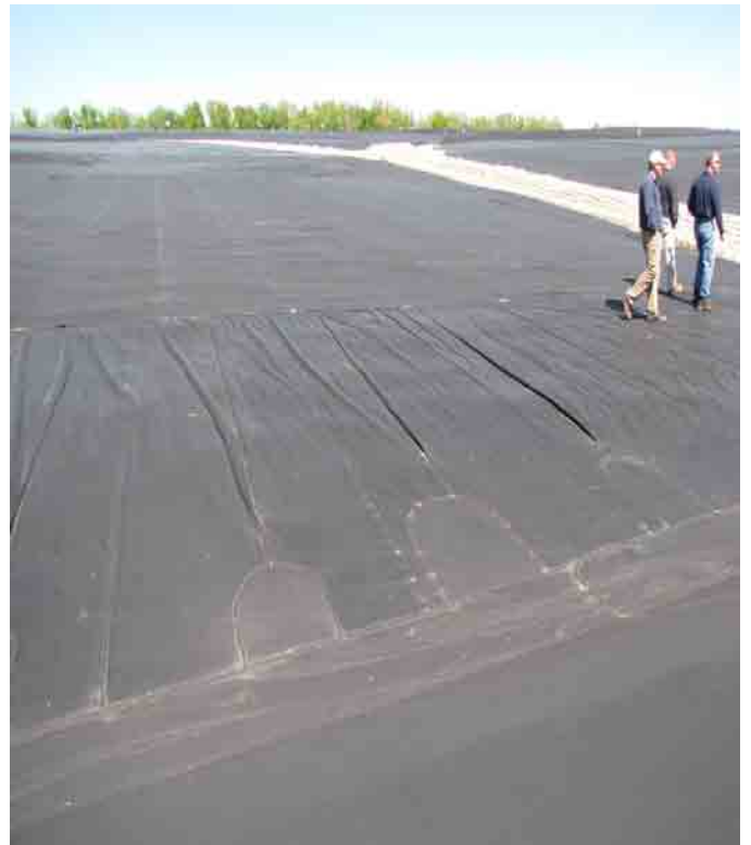
Interior diversion berm of interim cap, south of y-channel.
