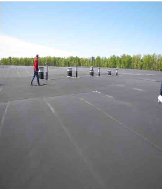
Top of previous leachate storage facility; Commonwealth access point to 20,000 stainless steel tank below.
