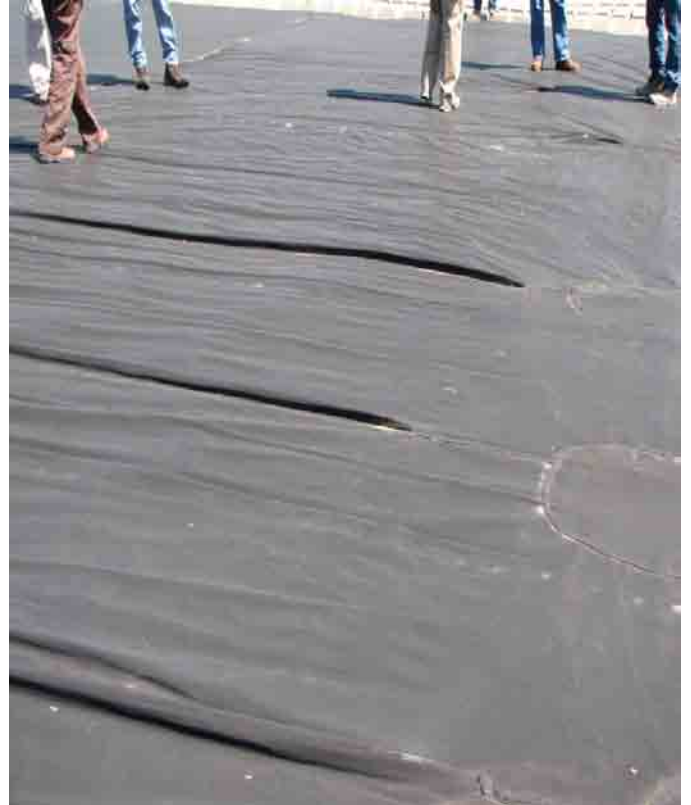
Interior diversion berm of interim cap, south of y-channel.
