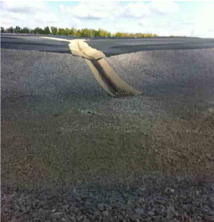
Outfall of Y Channel into East Detention Basin (EDB).
