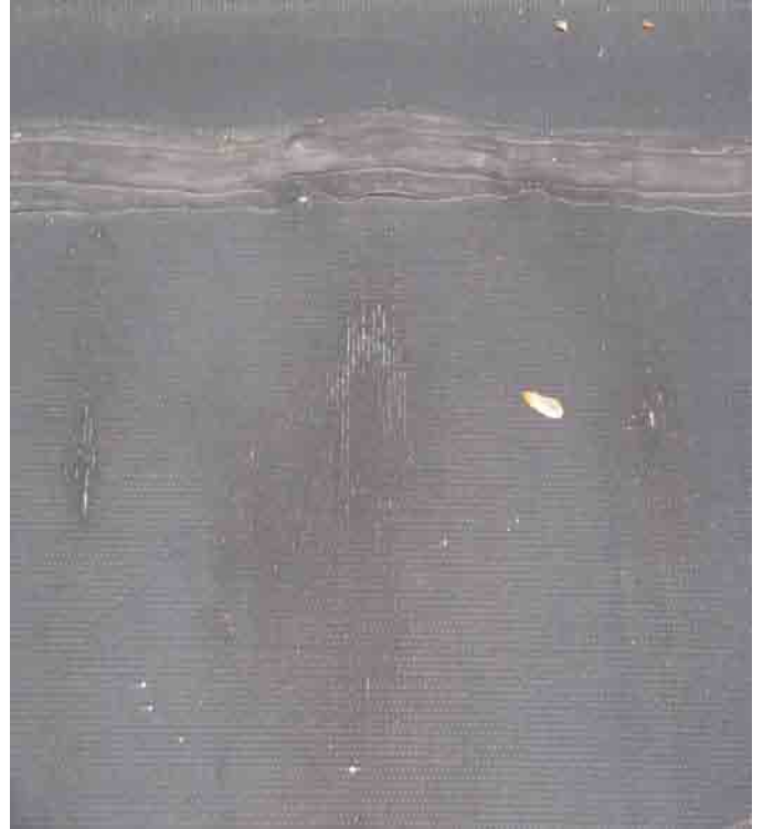
Close-up of liner striations on SW perimeter of interim cap.
