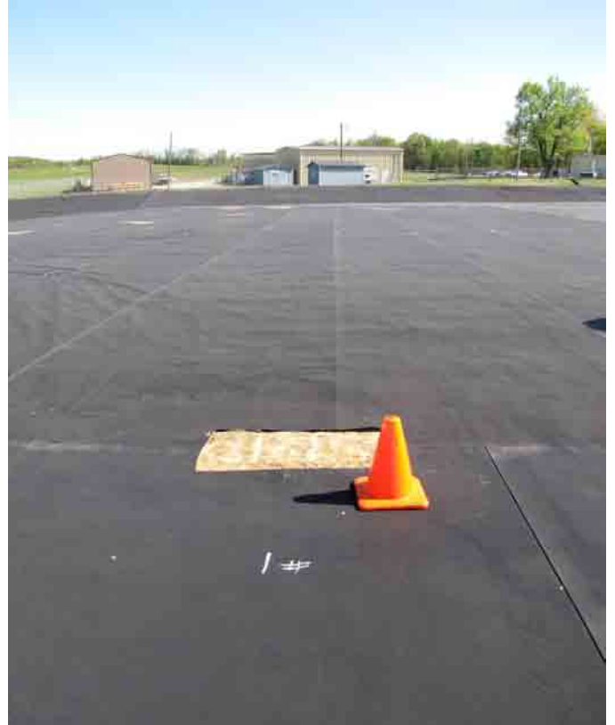
Independent liner inspection sample #1, looking north to Commonwealth buildings.
