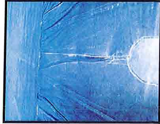
Typical Poor Quality Fusion Weld
