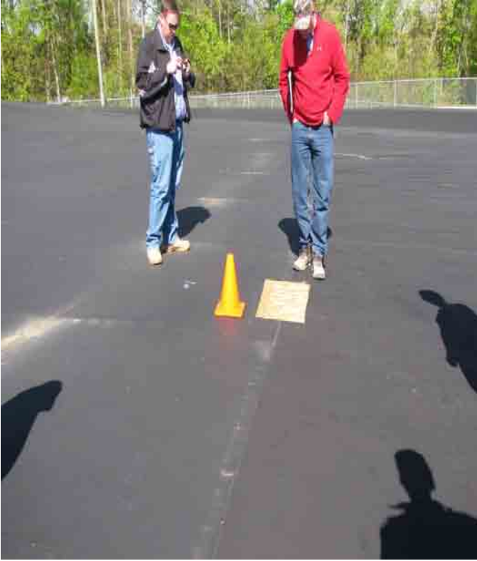
Independent liner inspection liner sample collection in northwest portion of interim cap.
