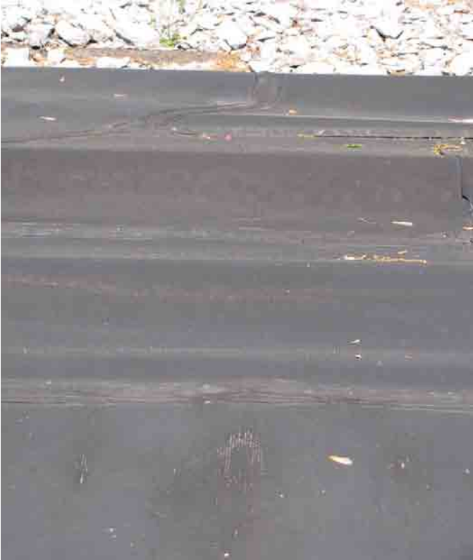
View of liner striation and anchor trench.
