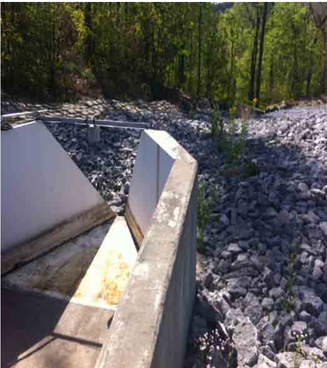
H-Flume looking in the East Main Drainage Channel (EMDC).
