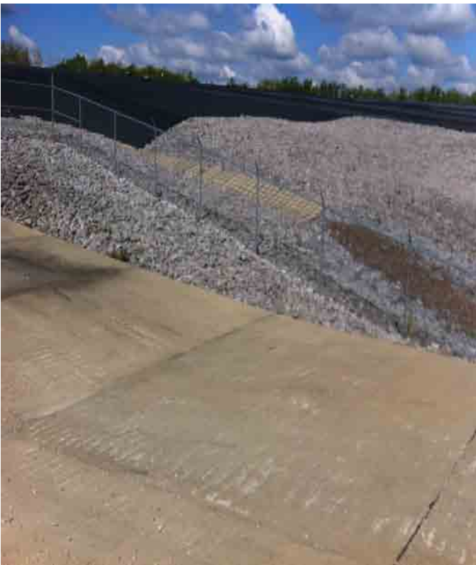
EDB emergency spillway.
