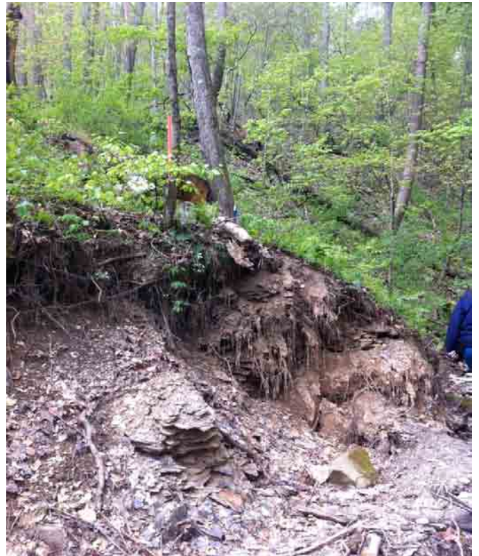
South bank near bottom of EMDC, note orange USGS survey marker.
