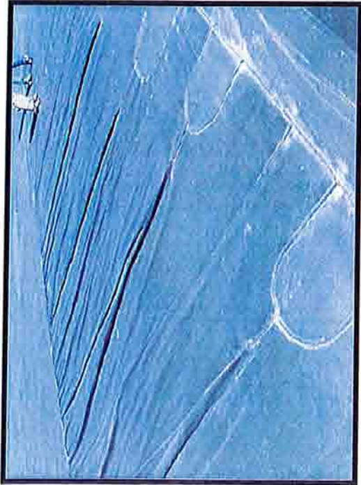
Typical Poor Quality Fusion Weld
