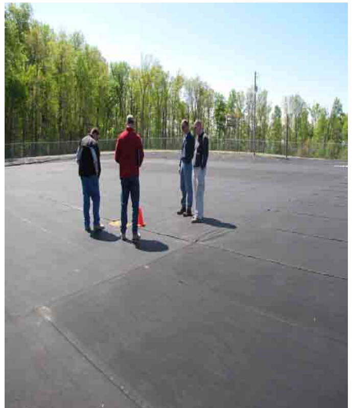
Independent liner sample collection in southwest portion of interim cap.
