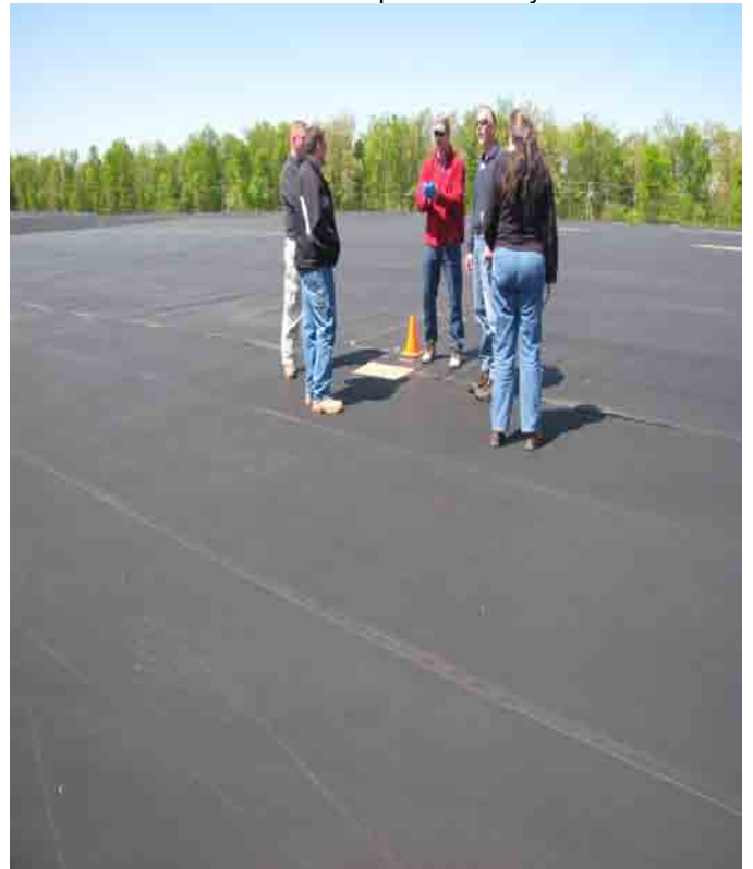
Independent liner inspection; liner sample collection.
