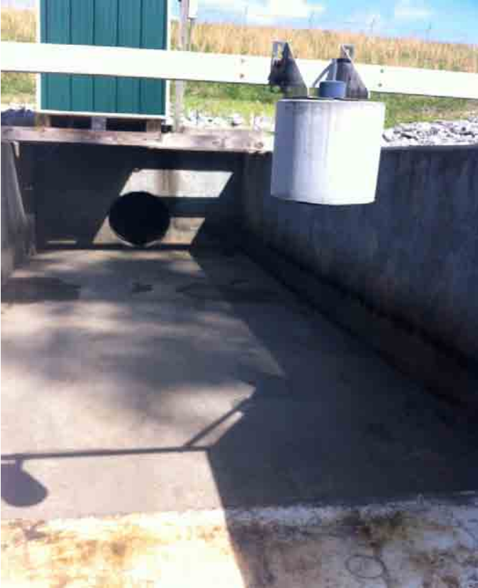
Inside of H-Flume.
