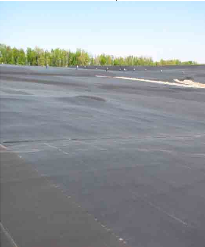
View of interim cap from southeast portion of liner; y-channel on right.
